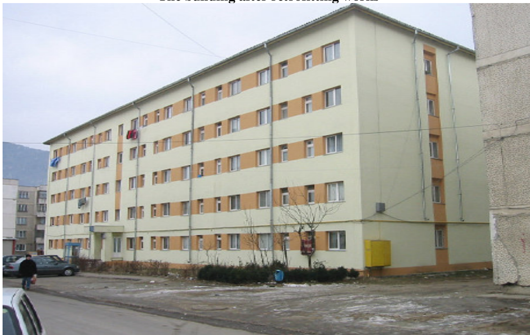
The building after retrofitting works
